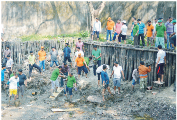
Cleaning of campus pond at Barrackpore
